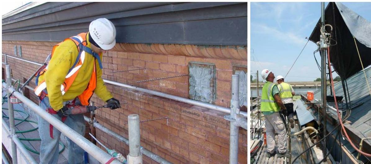
**Figure 7: At left, installation of helical wall ties into existing clay brick masonry walls. At right, coring at the top of the exterior walls in order to insert vertical reinforcing.**
