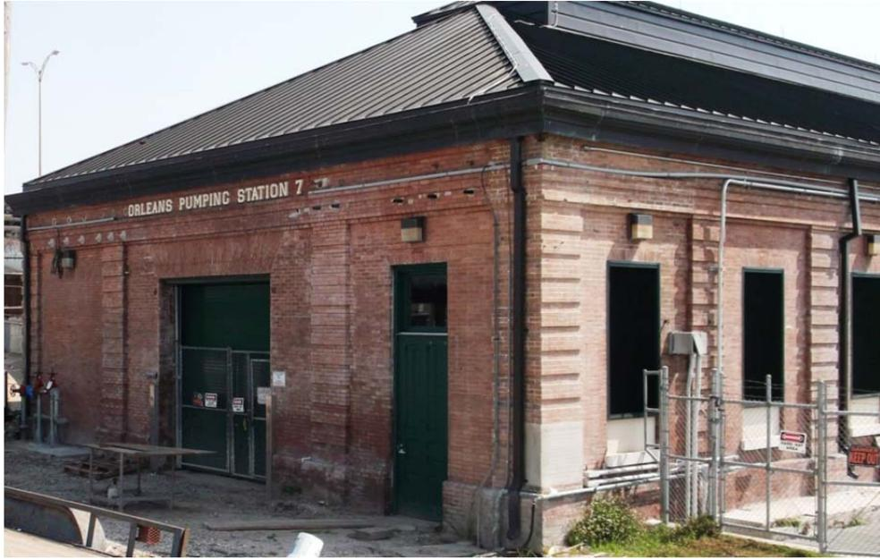
**Figure 10: Overall view of southwest corner of Drainage Pump Station Number 7 showing the clay brick masonry exterior walls after completion of the strengthening project.**
