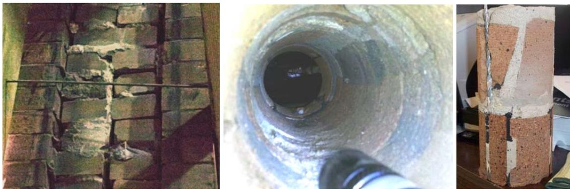
**Figure 11: Left, view of voids in brick masonry prior to injection at window jamb. Middle, view looking into a core hole made after completion of CIF injection showing the lighter colored CIF material has filled the voids in the wall. Right, core extracted from the exterior wall by the electrician after completion of CIF injection showing a helical wall tie and filled voids.**
