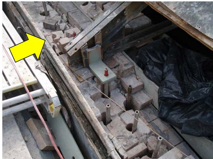
**Figure 8: Top of masonry wall condition during vertical reinforcing installation. Dislodged bricks are indicated with an arrow.**
