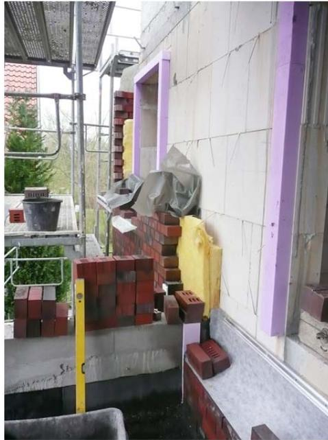
**Figure 2: Construction of masonry veneer walls, referring to fig. 1**
