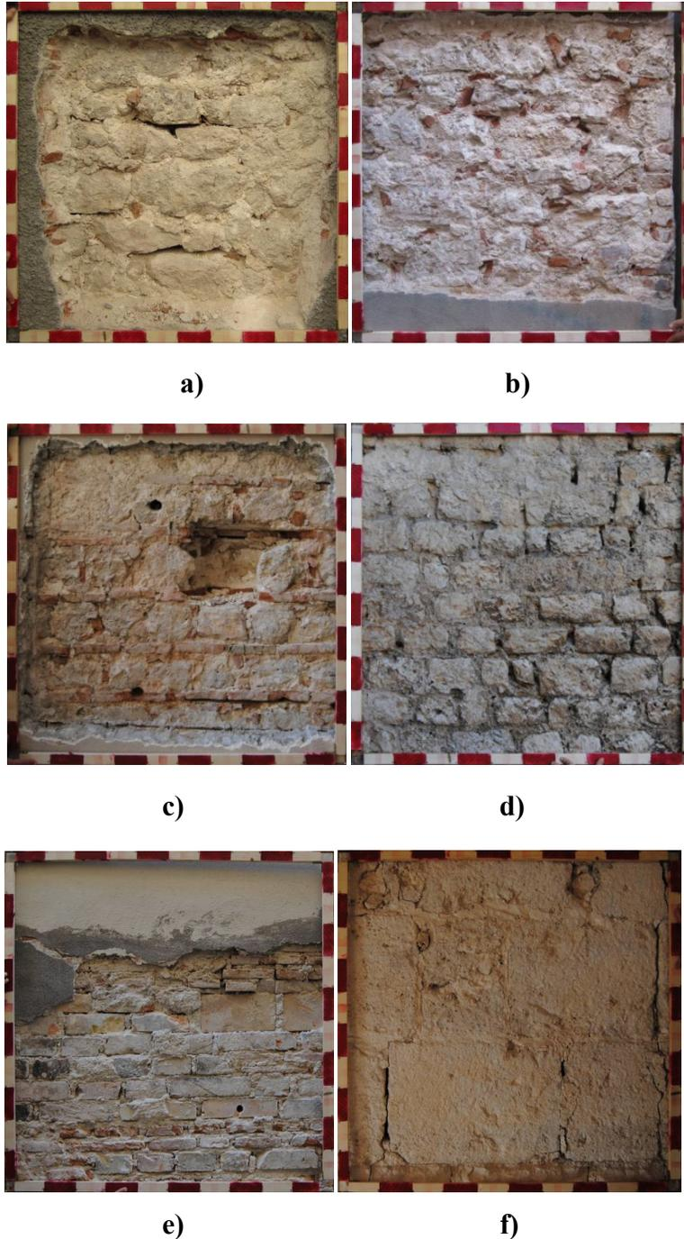
**Figure 1: L'Aquila's local masonry: a) irregular stone; b) irregular stone with brick pieces; c) irregular stones with brick lines; d) apparecchio murario aquilano; e) bricks; f) regular stones.**
