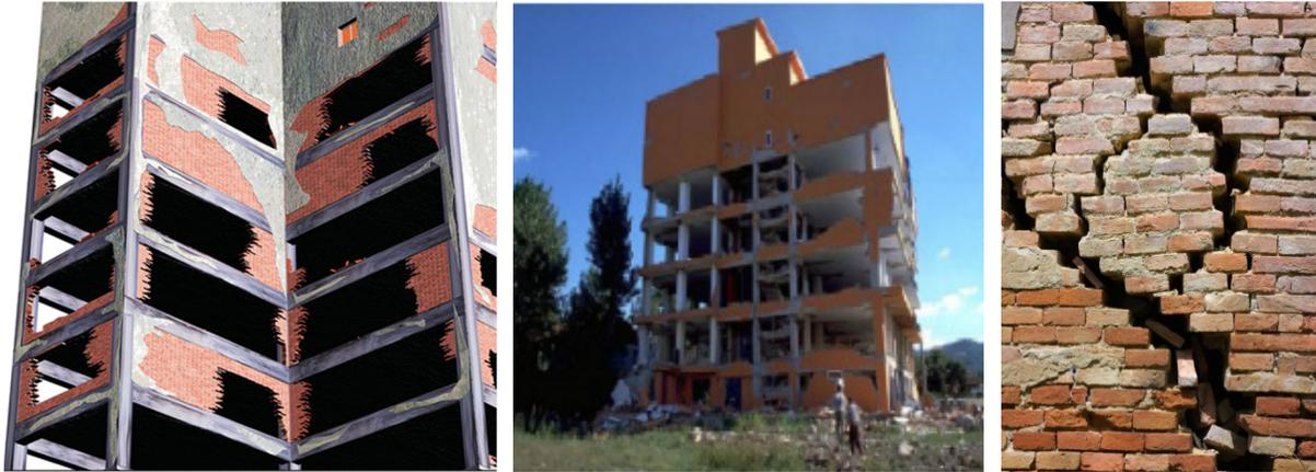
**Figure 1: Typical Damage to Masonry Infill Panels due to Earthquake Actions**
