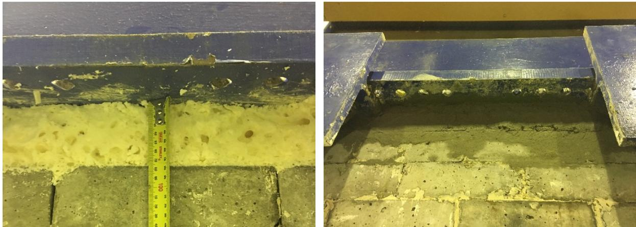
**Figure 4: Placement of Foam (left) and Grout (right)**
