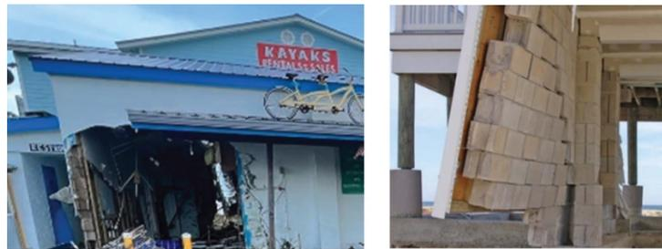
**Figure 1: Masonry wall failures during past storm surge events [4, 5].**
