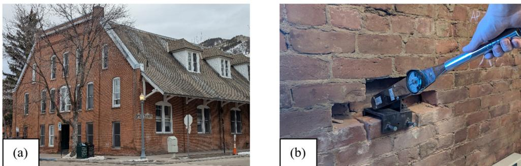
**Figure 7. Aspen Armory investigation: (a) Aspen Armory and (b) bond wrench testing.**
