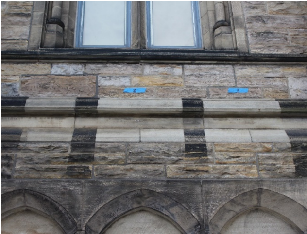
Proponent No.3: Mock-ups with Wellington Wall laser for assessment on CB
