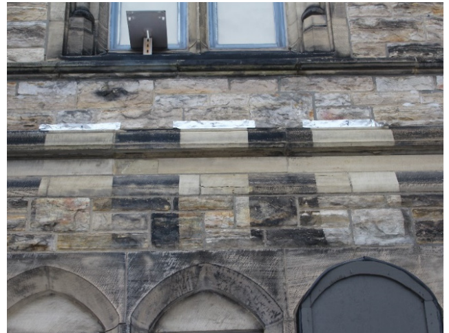
Proponent No.4: Mock-ups of East Block and Canada Four Corners contractor and laser for assessment on CB
