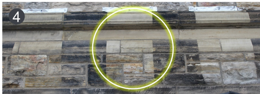
Proponent No.4: East Block and Canada Four Corners contractor and laser, selected by team, and considered acceptable level of clean
