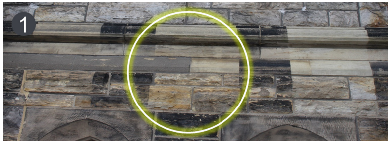
Proponent No.1: West Block contractor and laser, selected by team, and considered acceptable level of clean
