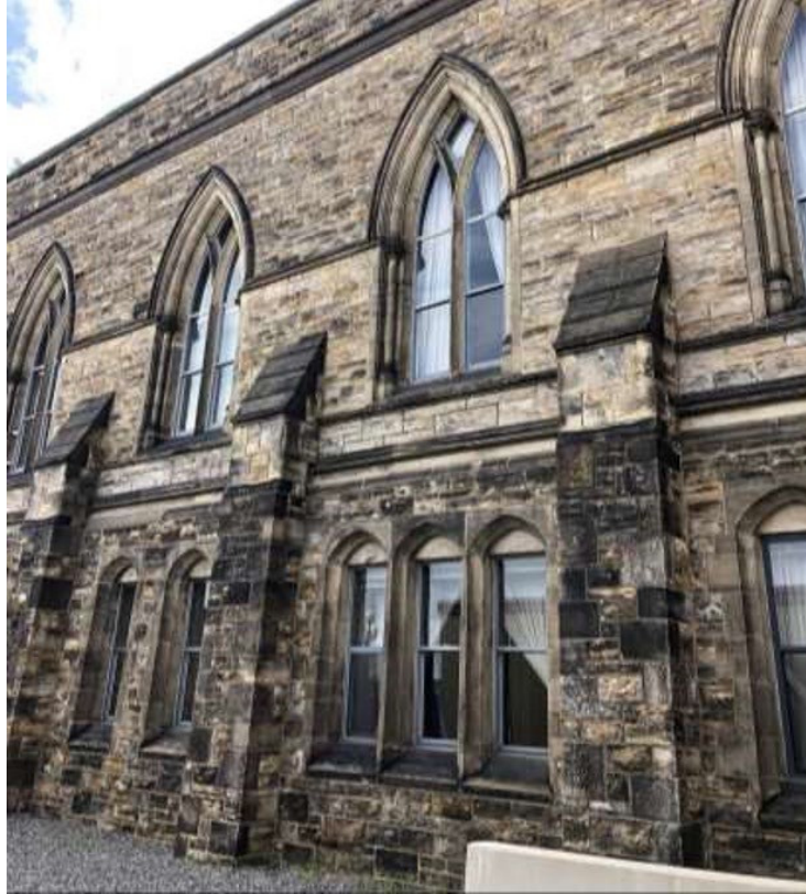
Nature of soiling on CB's exterior
