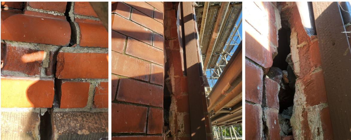
**Figure 7: Detachment of the outer wythe of the northwest tower.**
