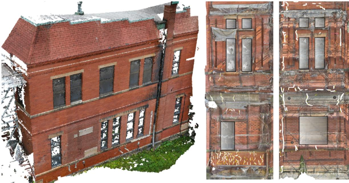
**Figure 1: (a) Photogrammetric model of the East façade of the building; (b) and (c) Damage mapping on the ortho-rectified photograph of the North and West faces of the northwest tower.**
