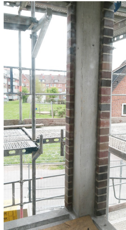
Figure 5: Standard construction practice with veneer walls; precast concrete element with thin brick veneer layer, as delivered to the construction site (left), and installed as load-bearing support (right)
