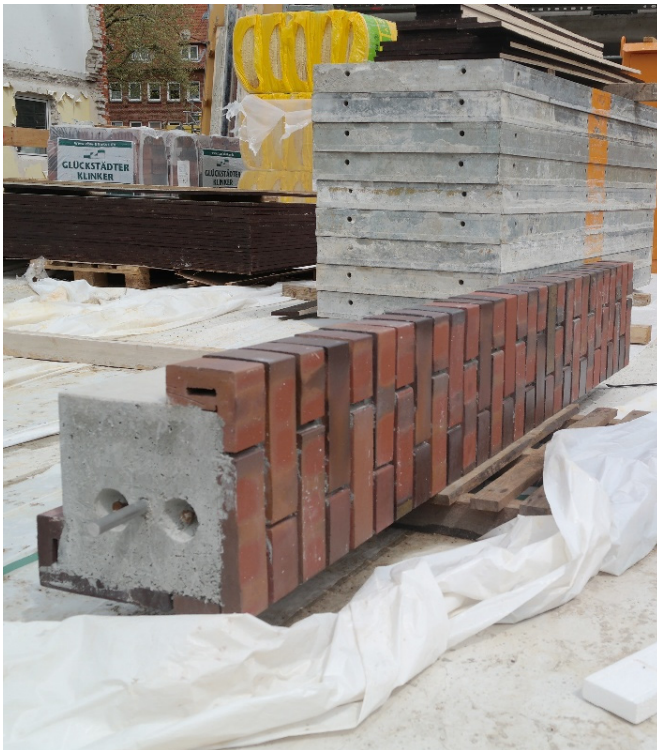
Figure 5: Standard construction practice with veneer walls; precast concrete element with thin brick veneer layer, as delivered to the construction site (left), and installed as load-bearing support (right)
