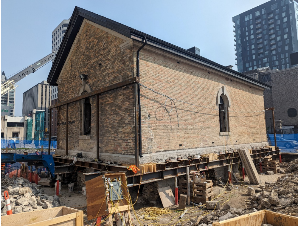
Figure 4: The steel platform partially installed, bearing on blocking and foundation [2023]
