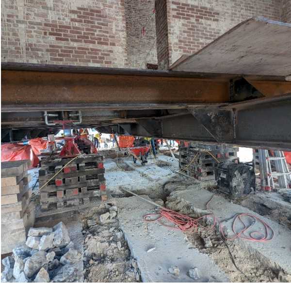
Figure 5a: Platform supported on jacks, foundation walls removed [2023]
