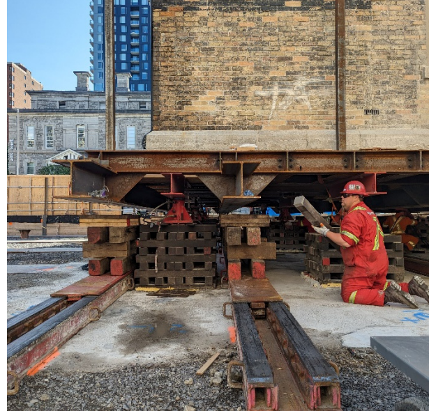
Figure 5b: Platform being lowered by jacks onto tracks [2023]
