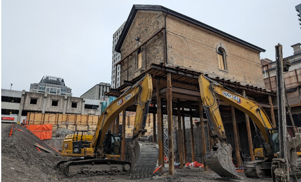
Figure 8: The CRO on piles during the excavation [2023]
