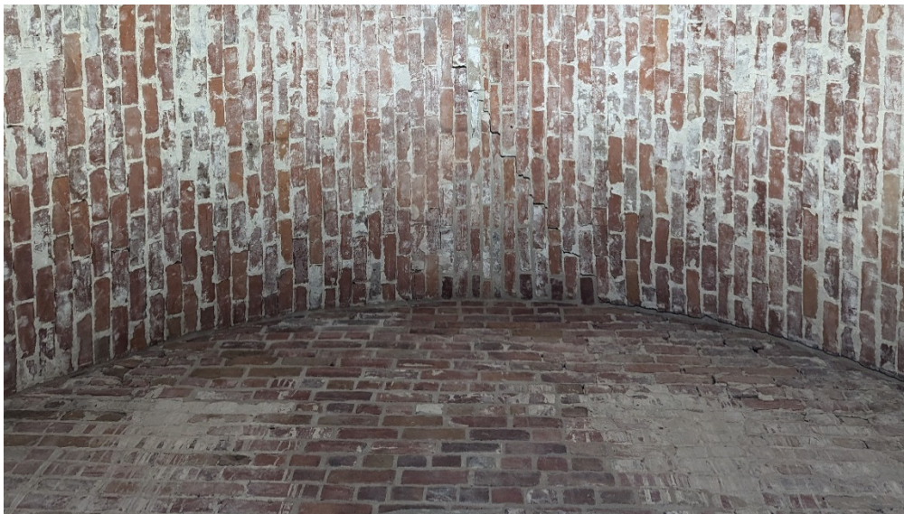
Figure 7: Cracking/separation of brick vault from perpendicular walls [2023]
