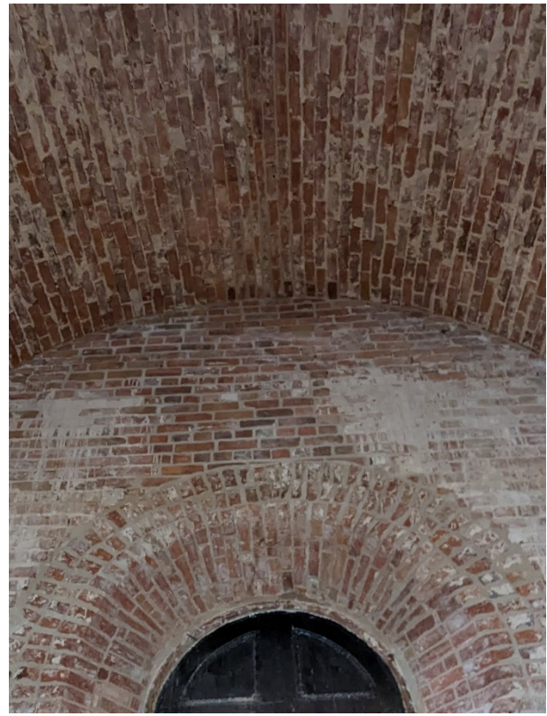
Figure 2b: Condition of the north wall, central room, after repairs [2022]
