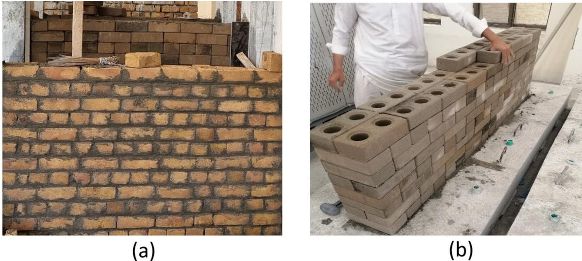
**Fig. 1. Masonry typology (a) traditional masonry wall (b) ICEB masonry wall under construction**
