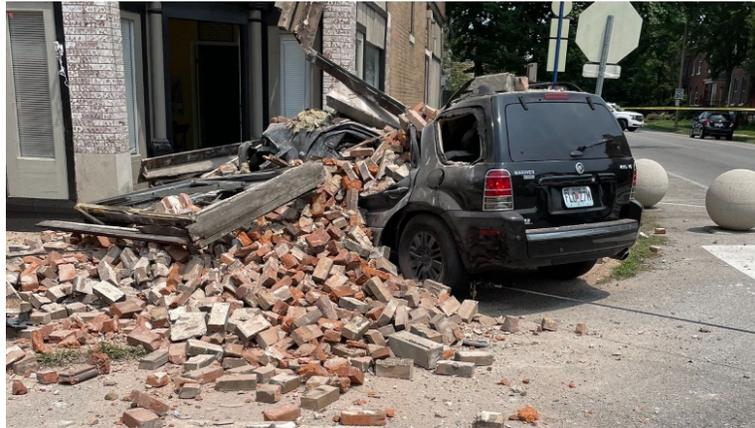
**Figure 1: Damage in the house due to vehicle impact.**
