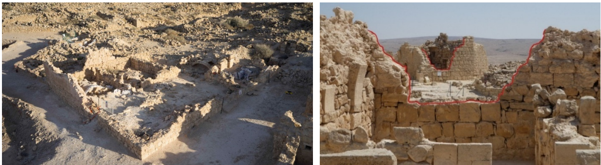
Figure 3: Aerial photo of building 86 (left). Collapsed masonry portion on the eastern side of the building and view of the Southern Church tower behind (right).
