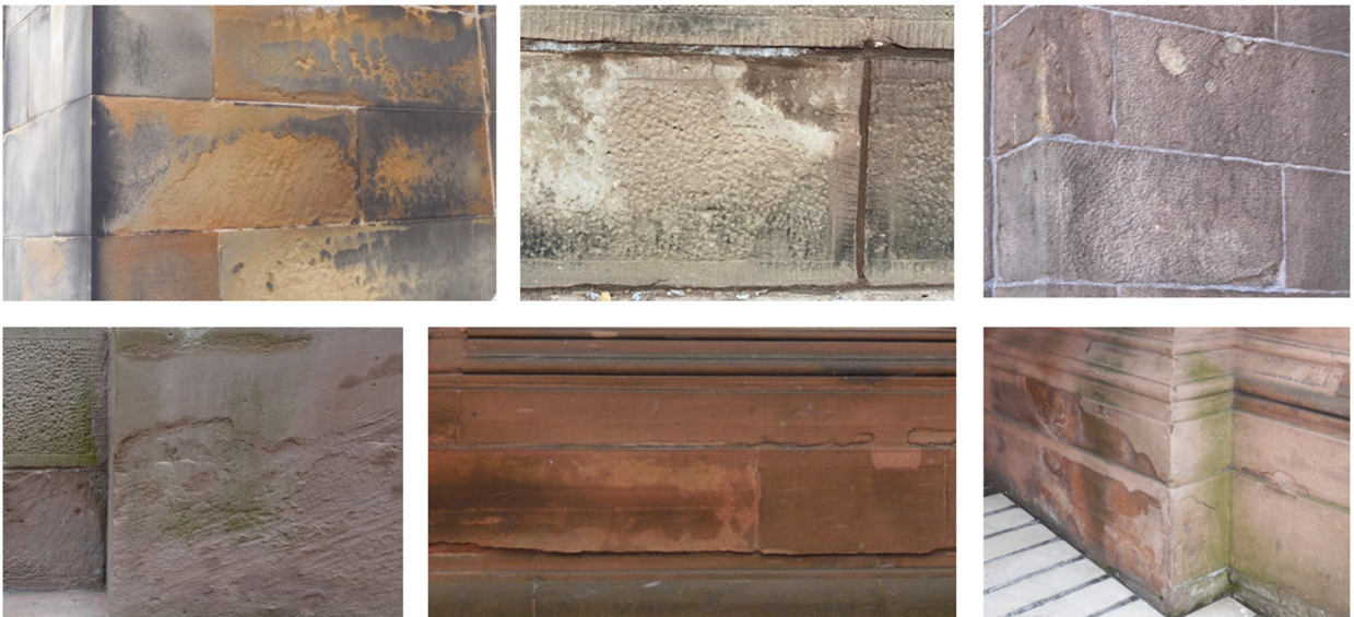
Figure 4: Examples of Sandstone in Fair Condition
