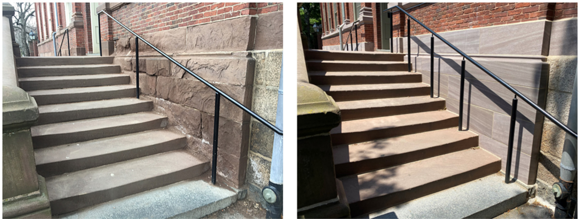
Figure 7: Replacing and Harvesting Stone at an Entire Architectural Element
