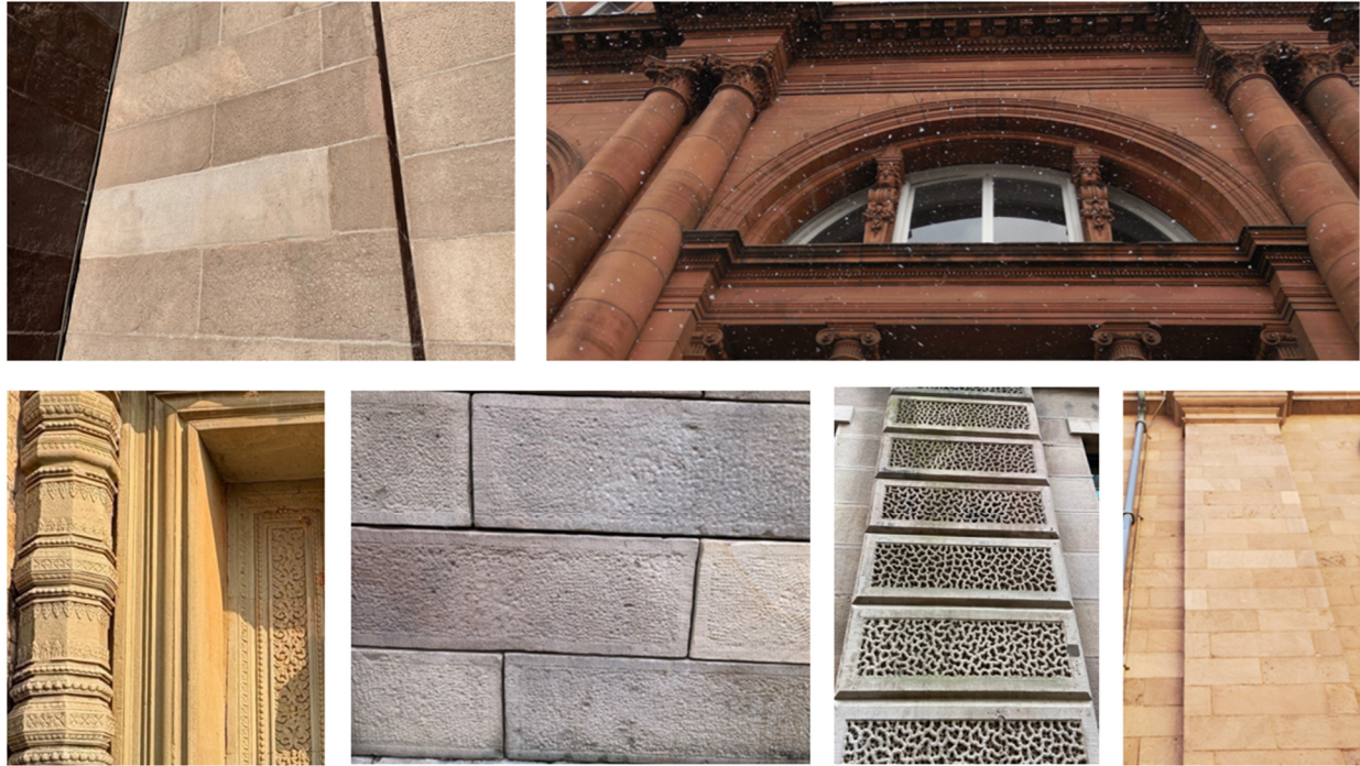
Figure 5: Examples of Sandstone in Good Condition
