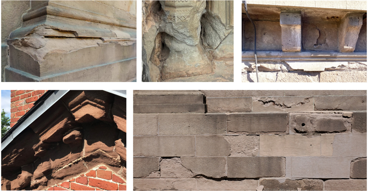
Figure 3: Examples of Sandstone in Poor Condition
