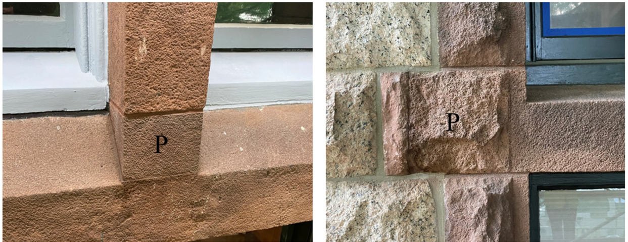
Figure 6: Example of Partial Stone Replacements Using Salvaged Original Stone
