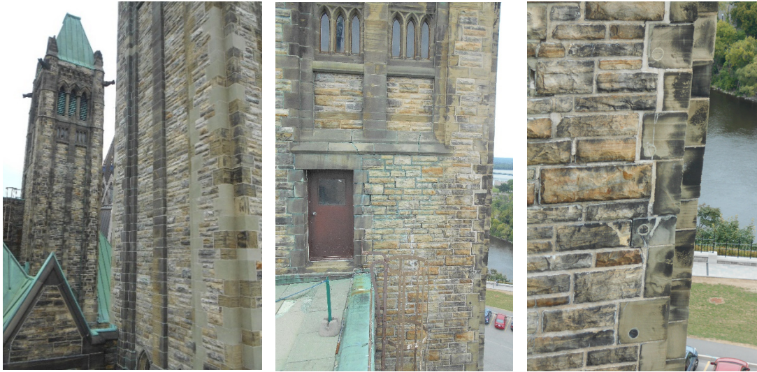
Figure 1: Conditions of towers in 2018. Left photo shows part of Tower 1 in foreground showing extensive stone replacement, and Tower 2 in the background. Centre and right photo show Tower 2 conditions
