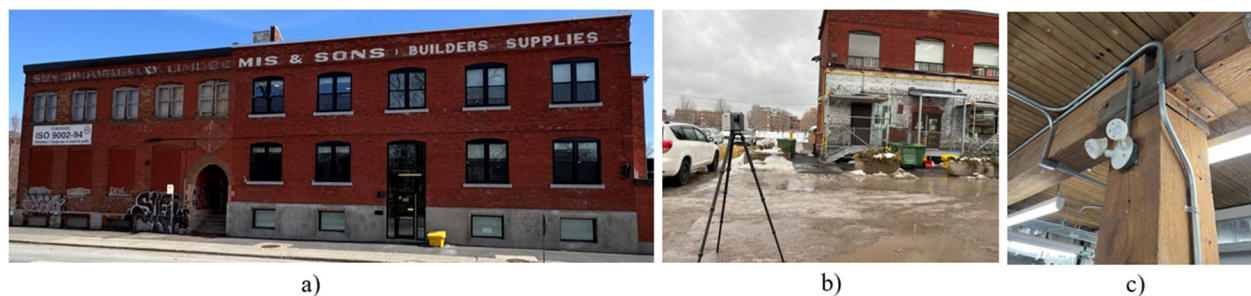
Figure 5: Rue Saint Patrick building a) street view b) laser scan and c) connection of the interior timber frame
