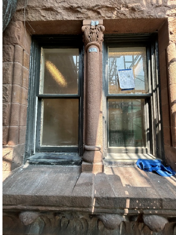
Figure 8: Vertical mullion between windows.
