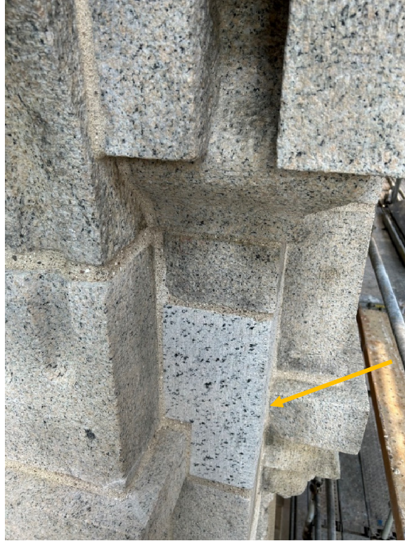
Figure 4: Milford Pink granite quarried in the early 1900s vs. 2000s (arrow).
