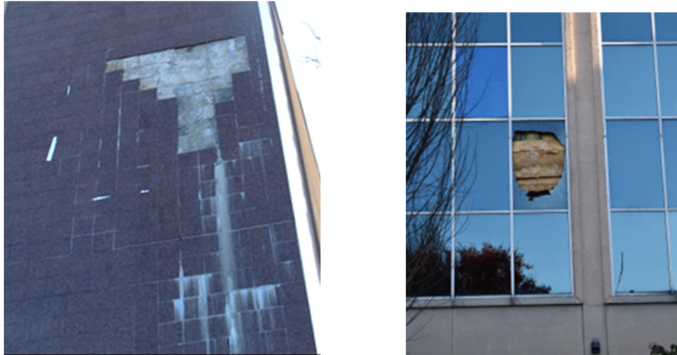
Figure 2: (a) Spalled granite tiles; (b) Broken glass
