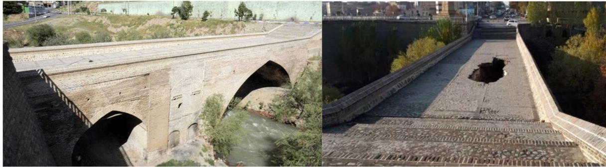
Figure 3: (a) Shah Abbasi Bridge; (b) Deck collapse in 2020
