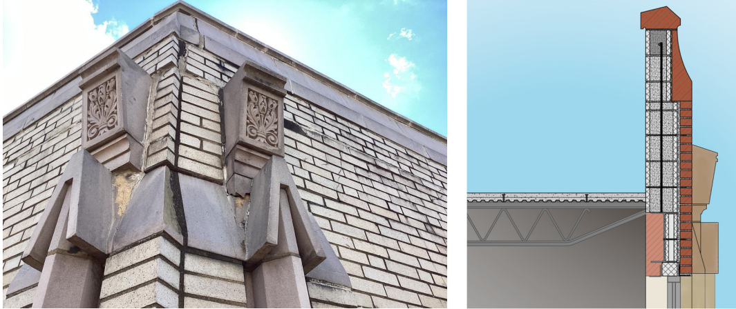
Figure 4: (a) Parapet damage; (b) Parapet repair section
