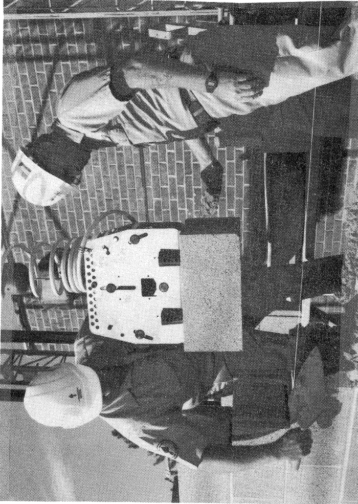
Fig. 4 A Two Man Crew can work Quickly and Efficiently with MAMA. Here, one bricklayer lowers a concrete block into position while the other loads his trowel with mortar.
